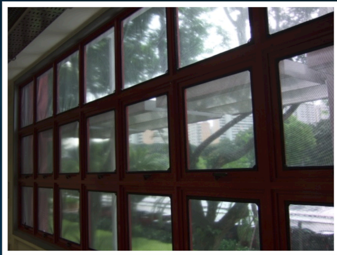
Inflector screen installed on single glass panes
