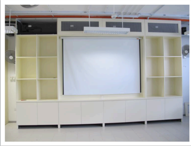
PDV installation at ZEB
