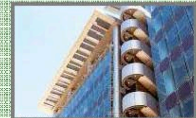
Solar Umbrella PV Systems for tropical rooftops
