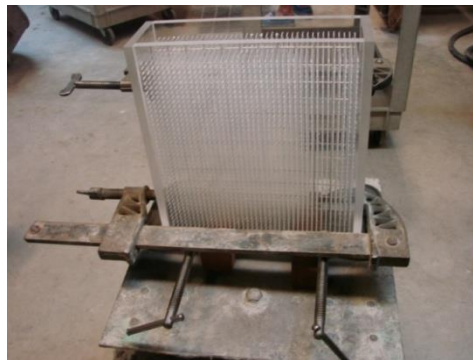
Before Mortar Placement
