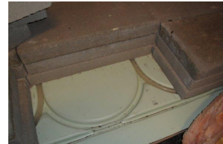
Real TABS construction
