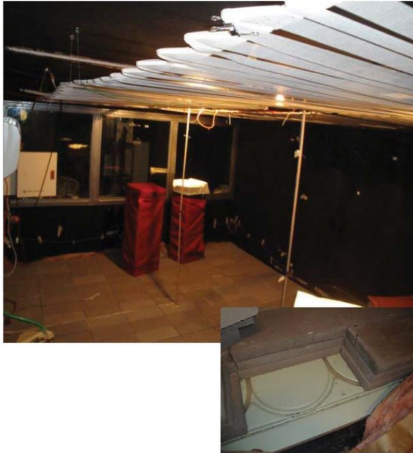
Radiant concrete floor
