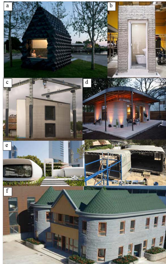
FIGURE 2 commercial projects printed (a) Micro-home printed in bioplastic in Amsterdam (b) Pre-fabricated bathroom unit printed in Singapore (c) 2-story house printed in Belgium in one piece (d) 3D printed single-story house in Texas (e) Printed office in Dubai (f) 2-story villa printed in China with reinforcements [12]–[16]
