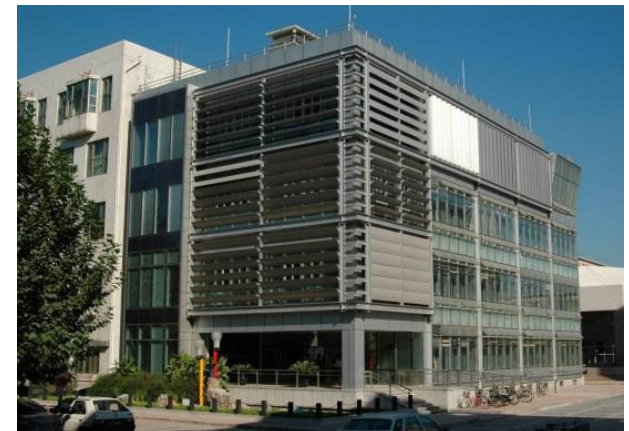
Low Energy Demo (LED) building @ Tsinghua
